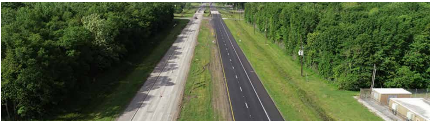
PHOTO DURING CONSTRUCTION OF LA 22 REHABILITATION PROJECT
